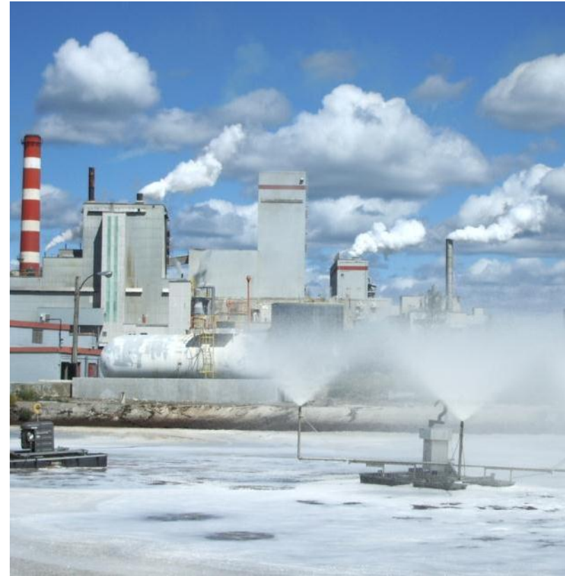
Energy efficiency upgrade to effluent treatment at Canfor Pulp
